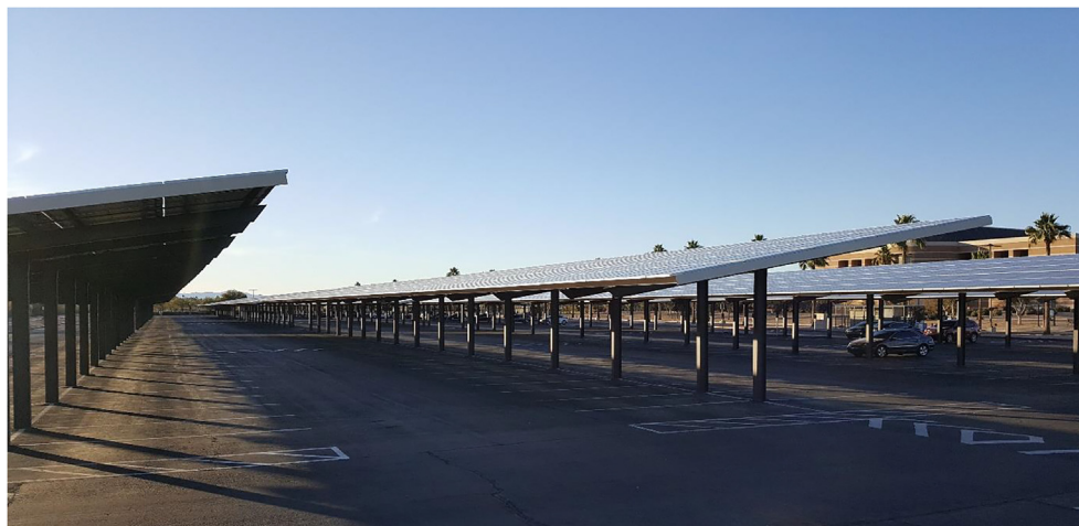
Fig. 7. Rows of PV shade structures provide shaded parking for hundreds of parking spaces on the Arizona State University west campus in Glendale, AZ. Photo: David Sailor.
