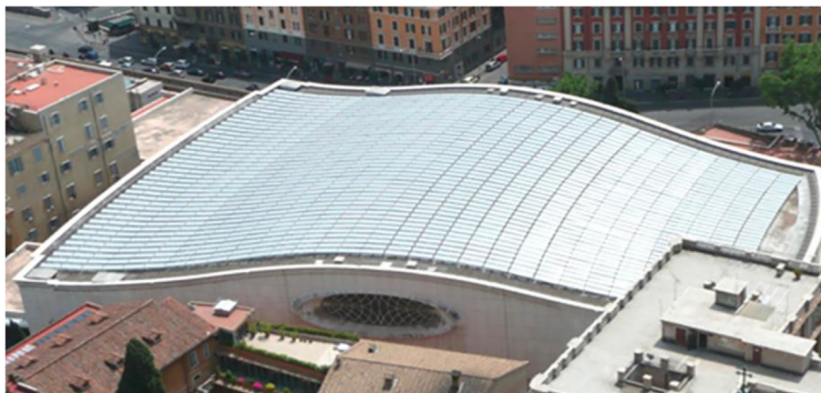
Fig. 2. A rooftop building-integrated photovoltaic (BIPV) system on the Aula Pierluigi Nervi, Vatican. Although the modules are on metal supports that are separate from the building structure itself, the array of modules has been aesthetically integrated into the architectural form.
