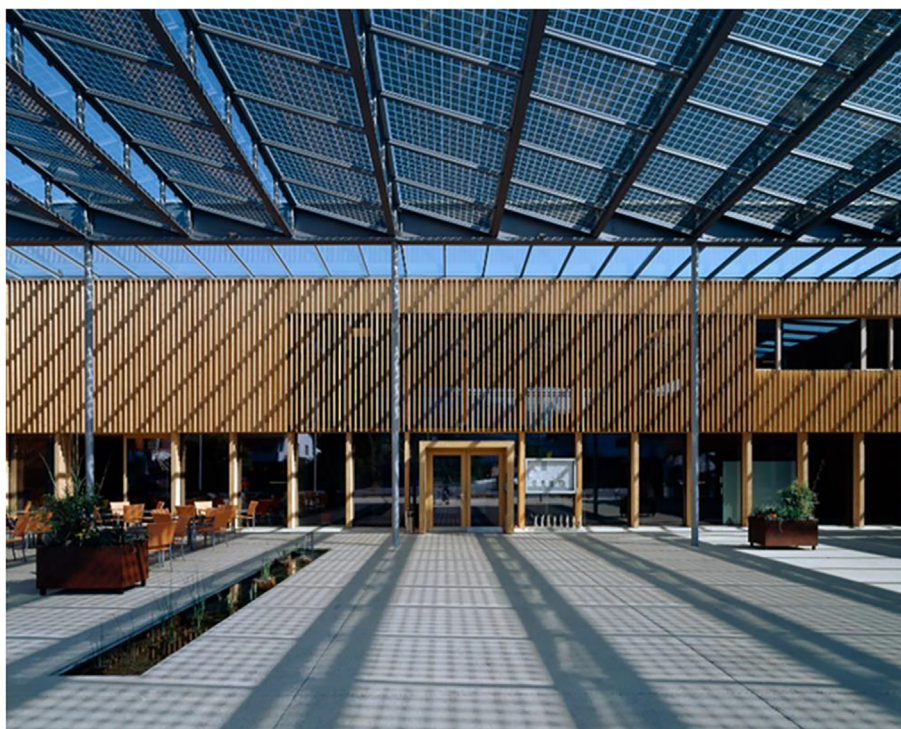
Fig. 3. Building-integrated PV providing solar electricity and shade for inhabited spaces at the Ludesch Community Center, Ludesch, Austria. Photo: Bruno Klomfar.
